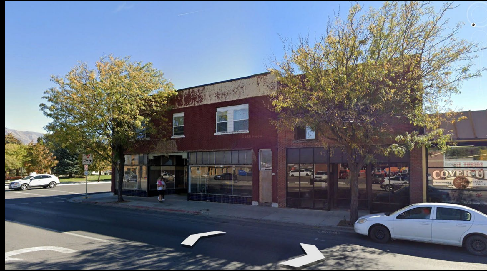
After removing the front facade exposing the original architectural details
