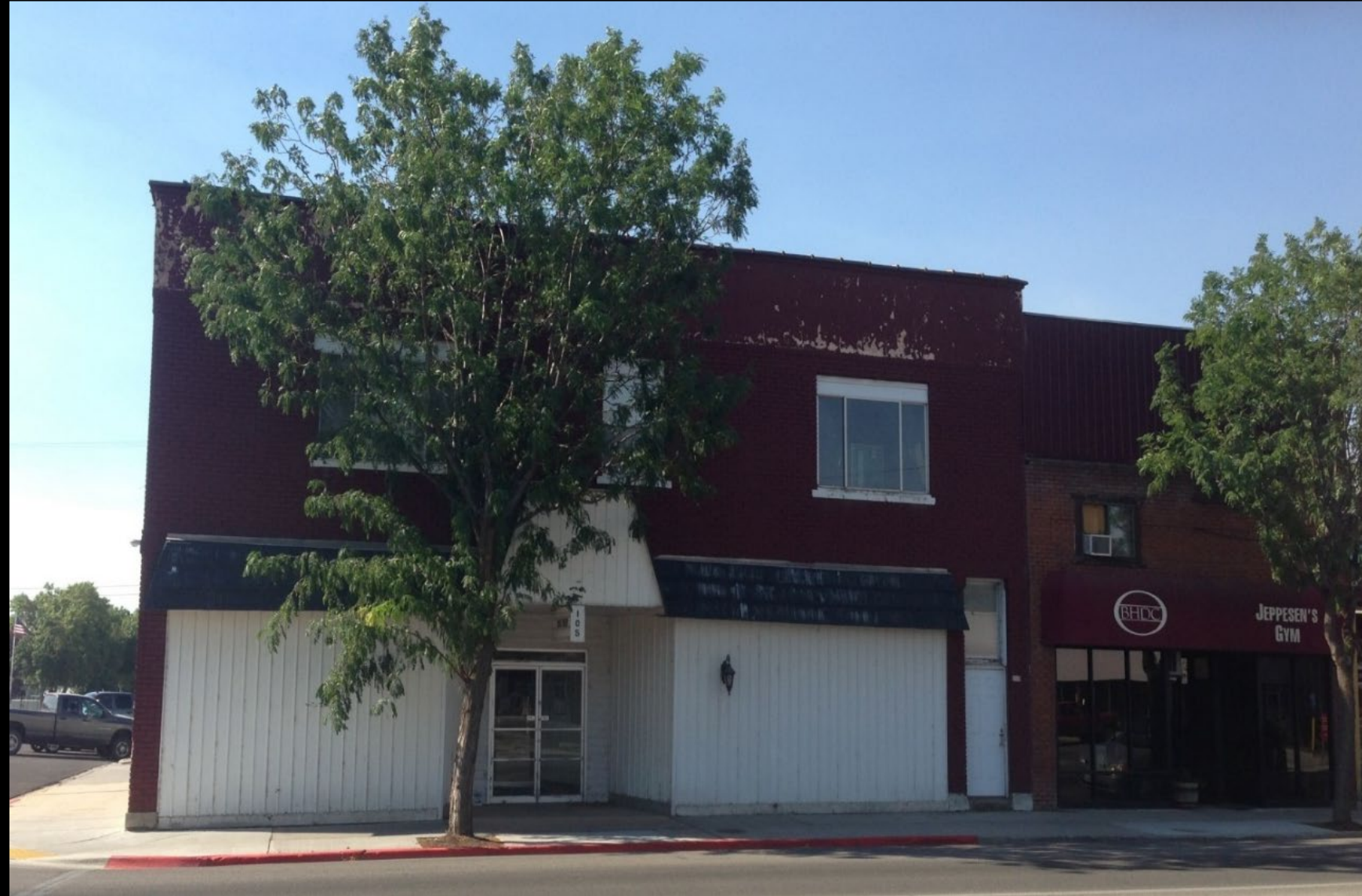
Before removing the front facade
