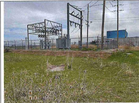
Subject Property Looking Southwest
