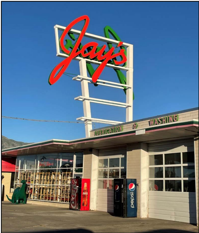
After- Jay's sign.
