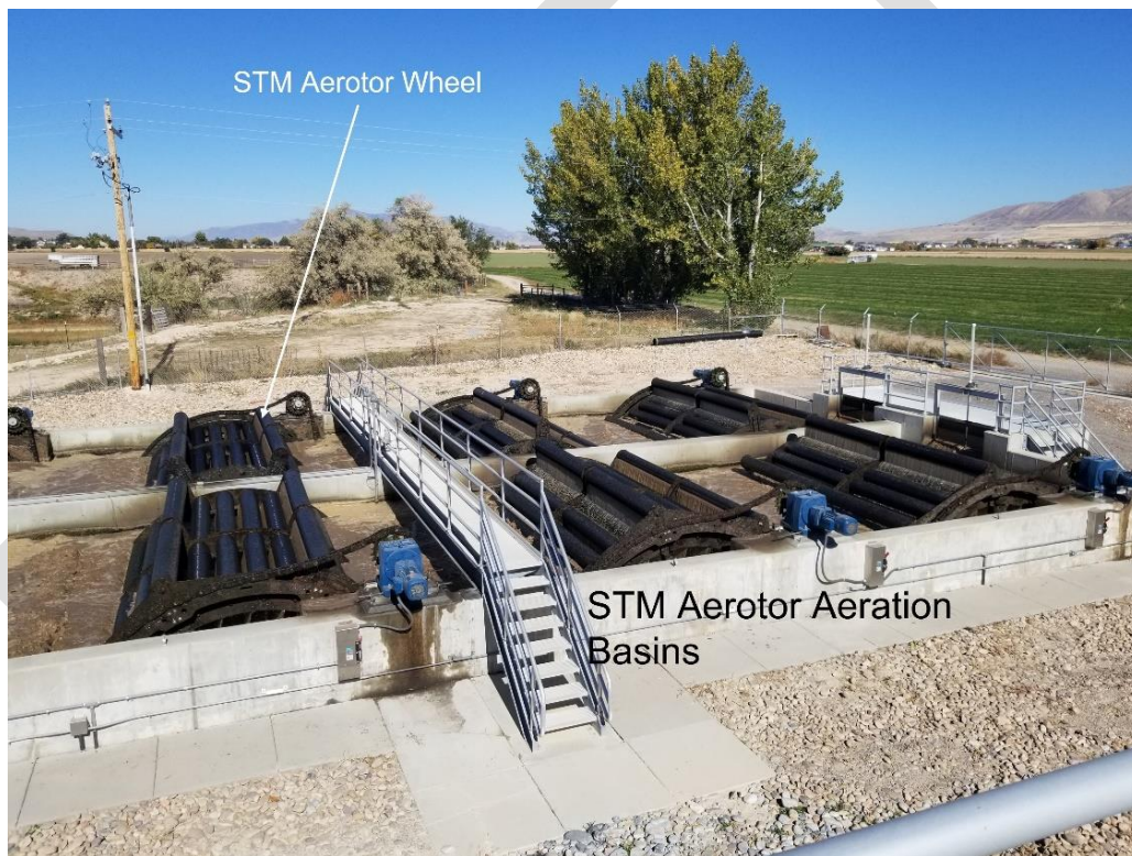
Figure 3-9: STM Aerotor basins.
