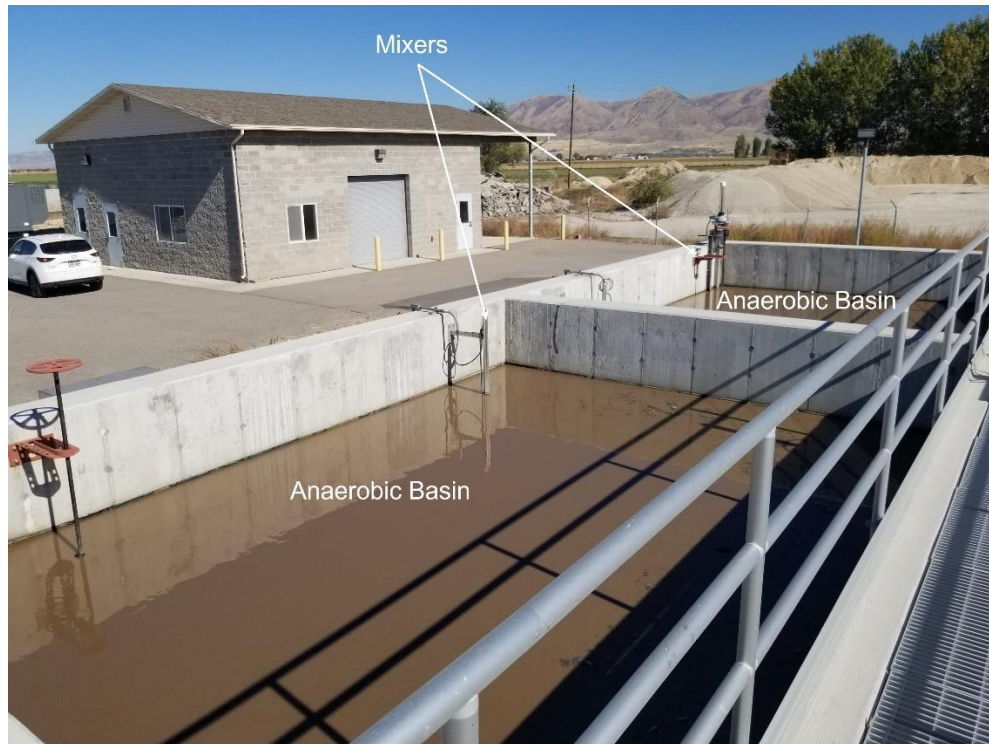
Figure 3-6: Anaerobic basins.
