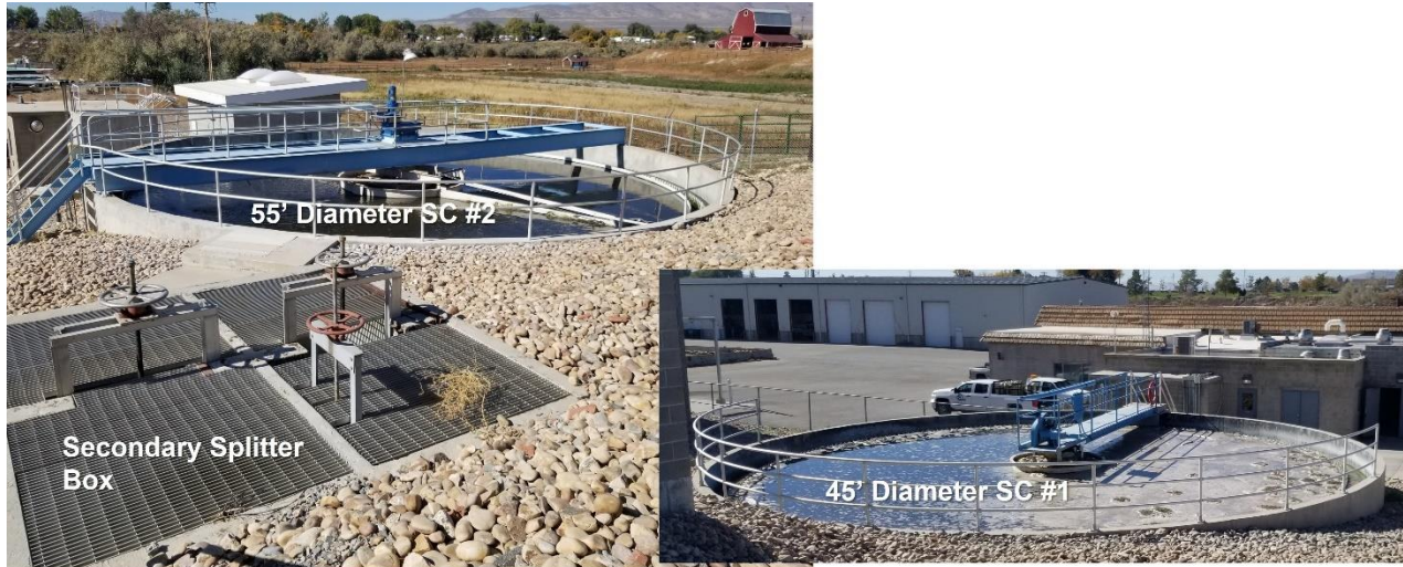
Figure 3-10: Secondary clarifiers.
