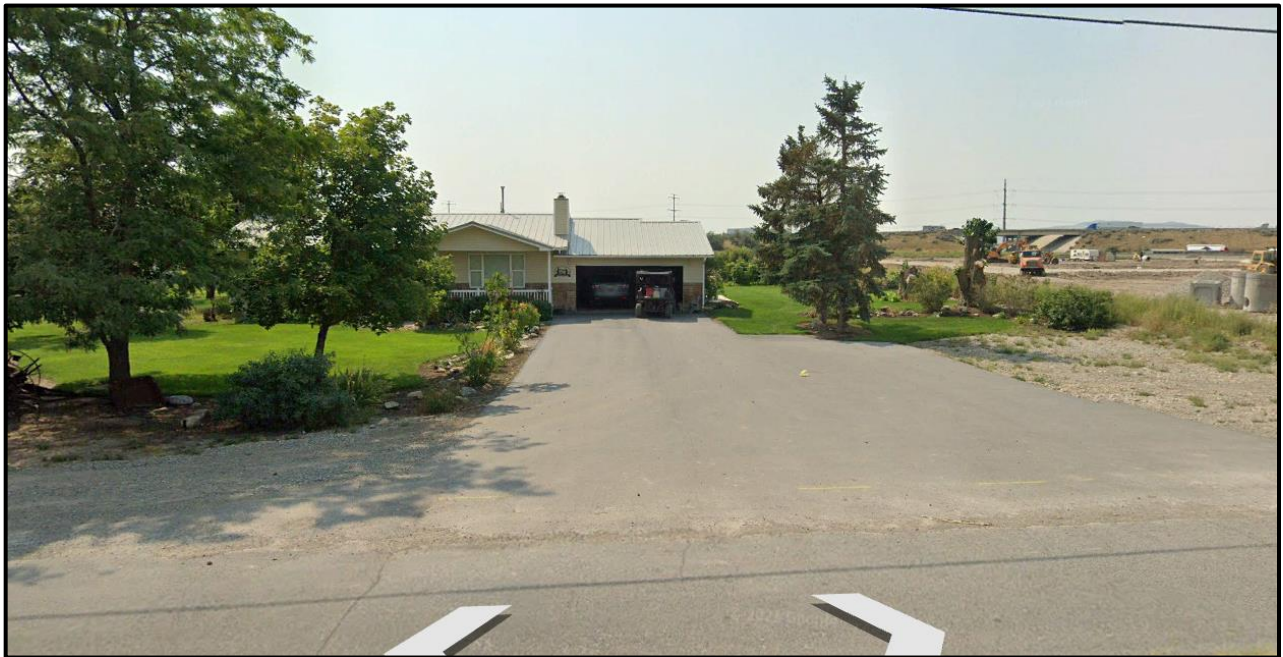
Asphalted Driveway on Parcel No. 05-200-0002
