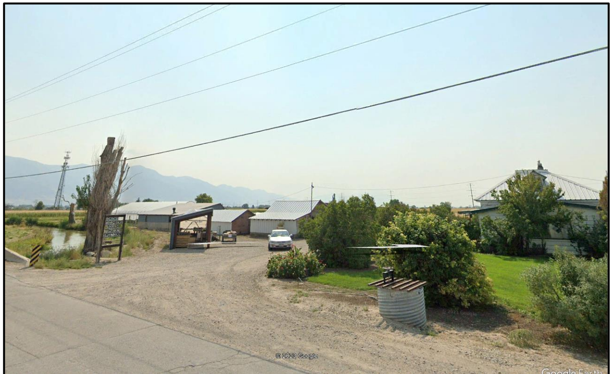
Irrigation Headgates on Parcel 05-200-0003
