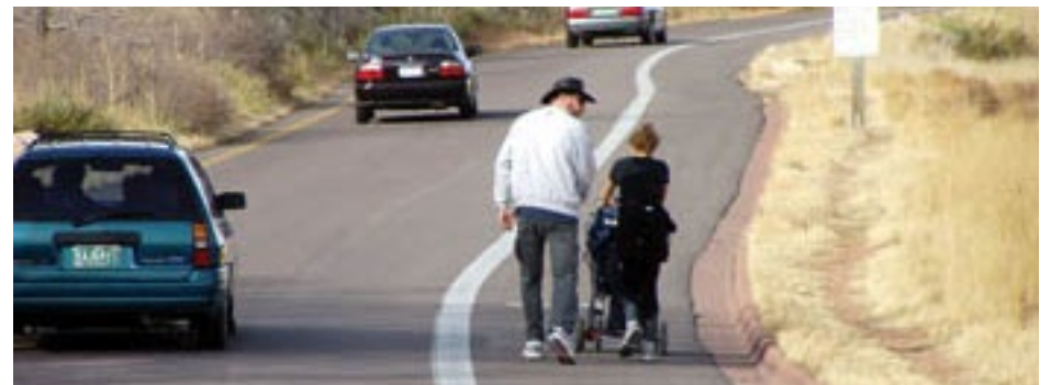
This extra thick white stripe reduces the lane size and protects the pedestrians.
