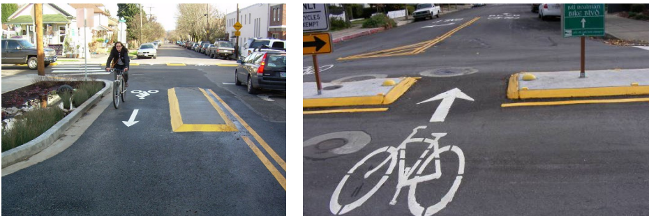
Streets are converted to bike boulevards with signage, striping and minimal medians.
