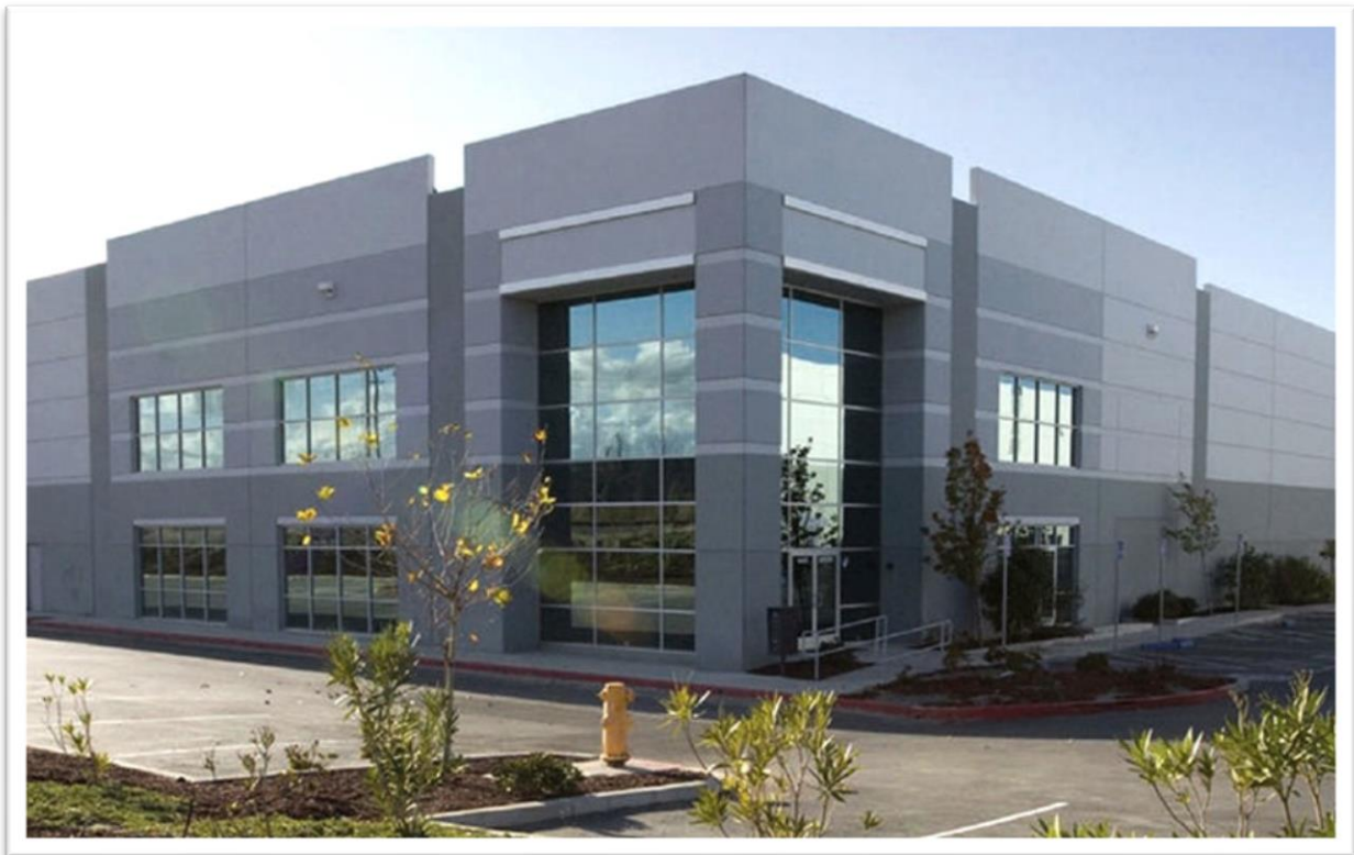
Picture of typical flex office building
